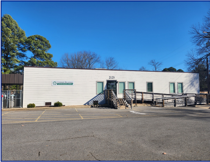
View of subject property facing E
