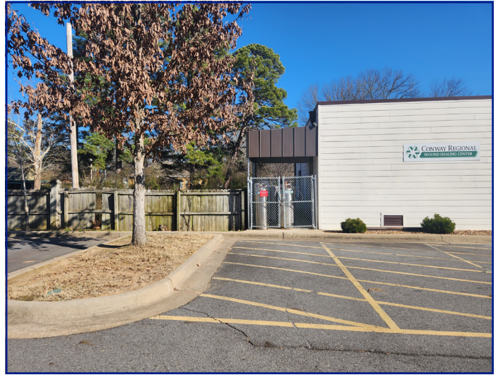
View of subject property facing E
