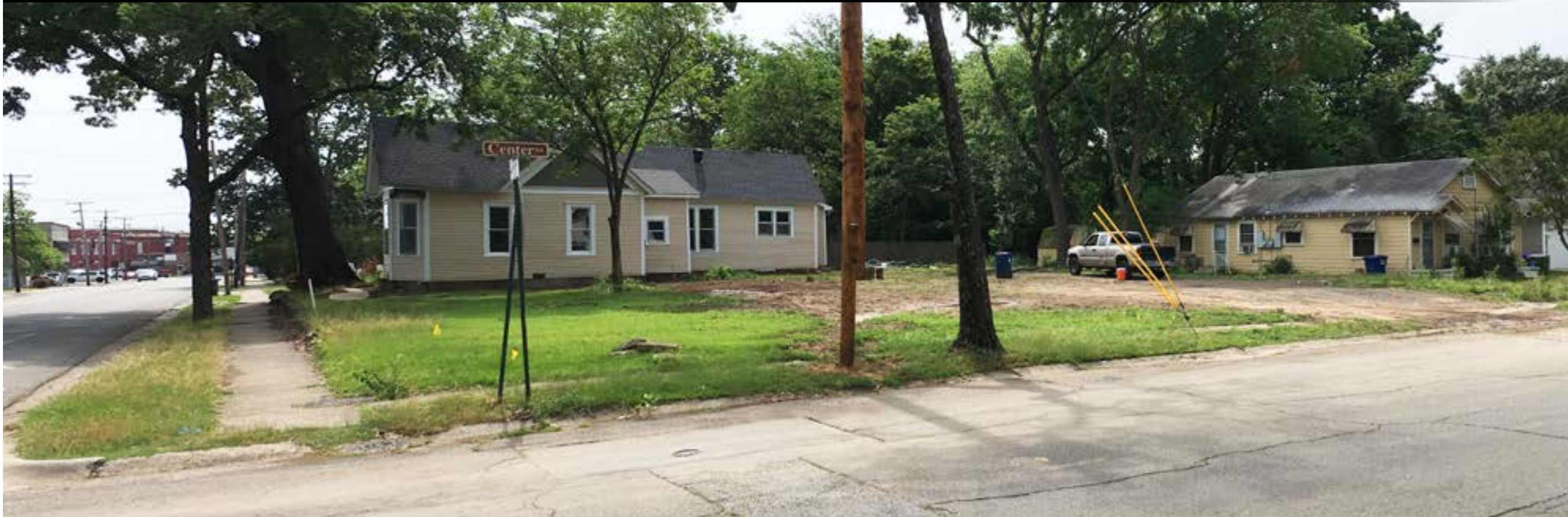
View of property from Center St looking E
