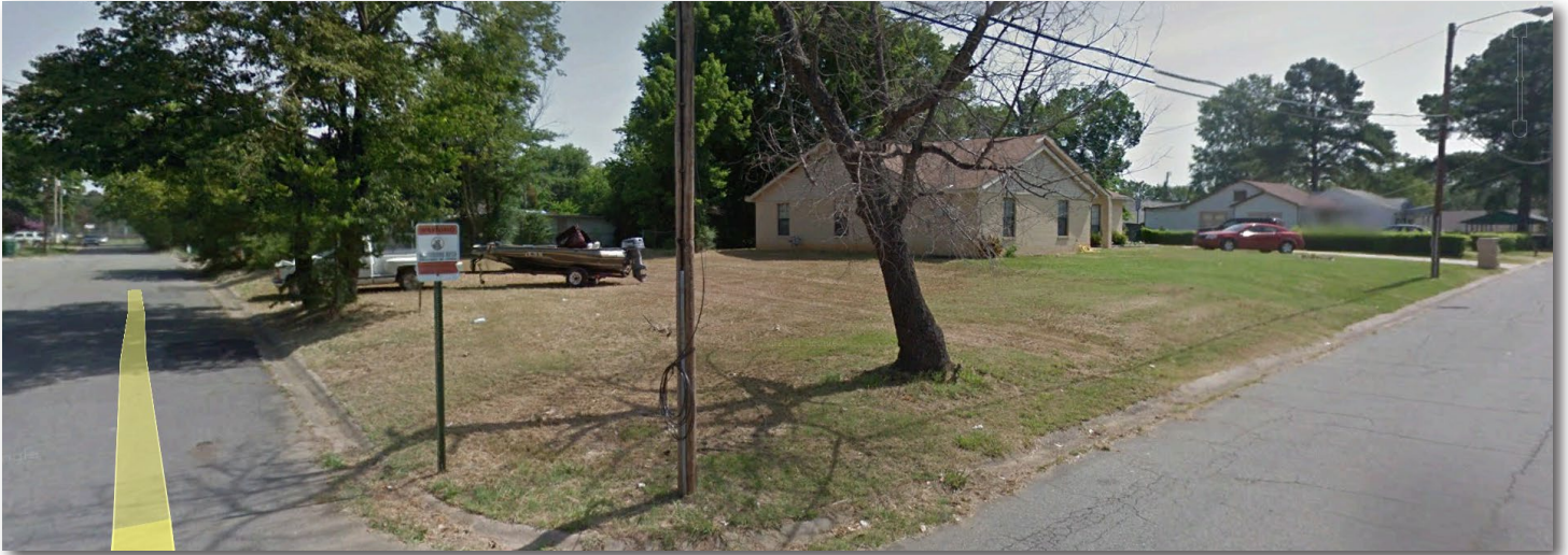
View of 716 Pine Street looking NE
