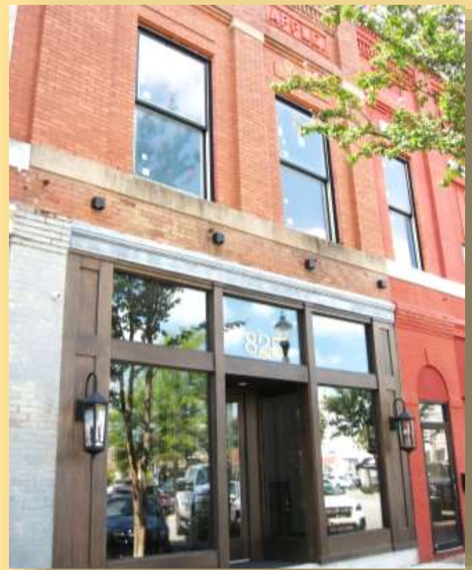
Recent tax credit project - 825 Parkway Street.
