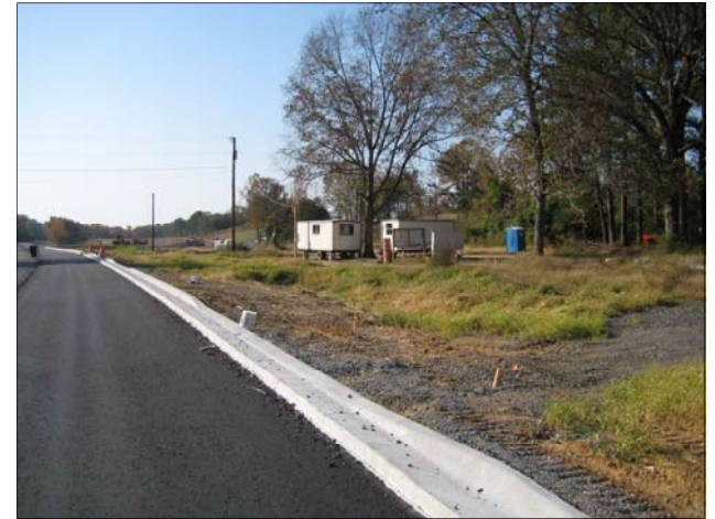
Installation of curbs along newly widened portion of Old Morrilton Highway.
