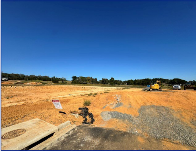
View of subject property looking NE
