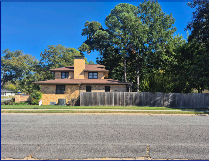
View of subject property facing E
