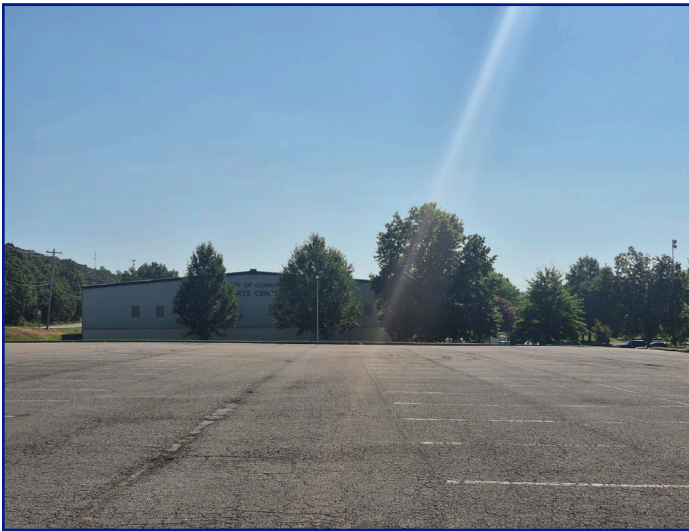
Primary structure on site
