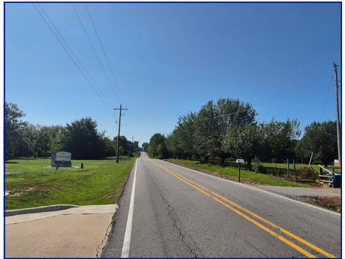
View along Skunk Hollow Rd facing S
