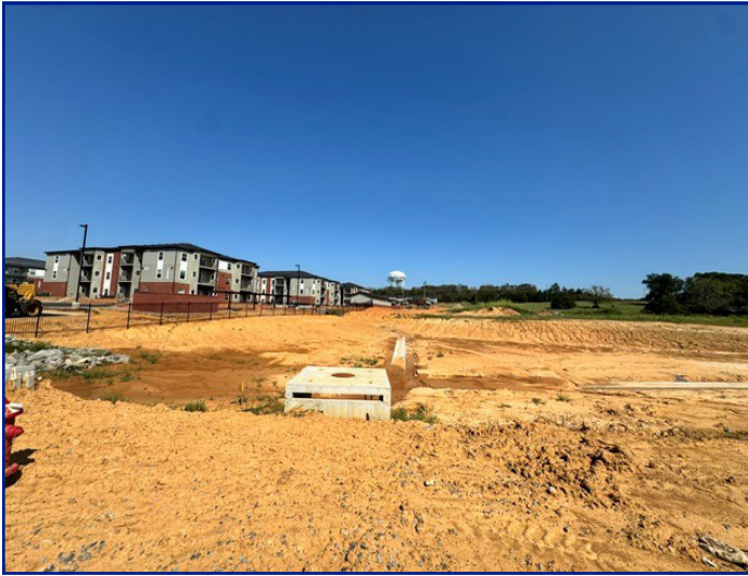
View of subject property facing N
