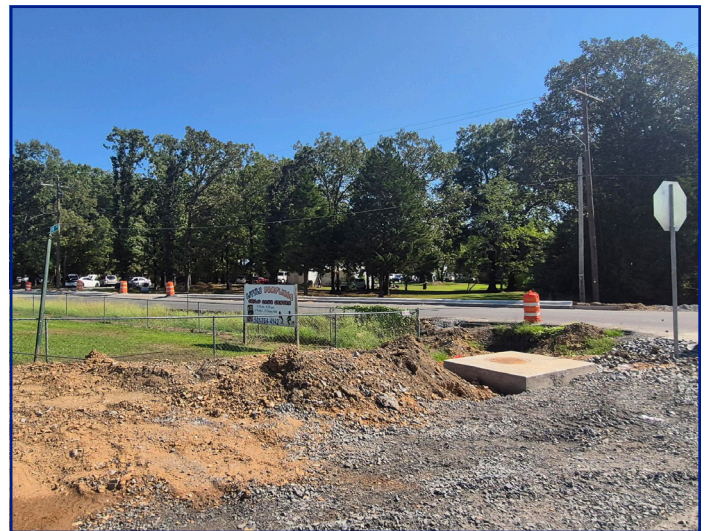
Intersection of DWD and Skunk Hollow Rd
