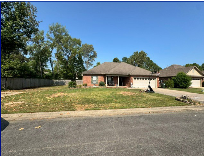
Adjacent property to the NW
