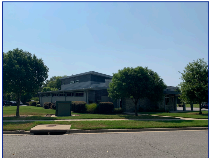
Adjacent property to the E
