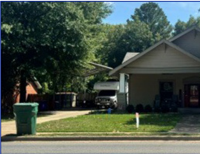
View of carport on subject property
