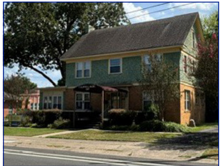
Adjacent property to the E
