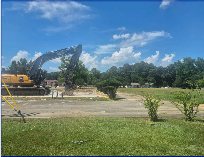
View of subject property from Silver Springs Cir facing N
