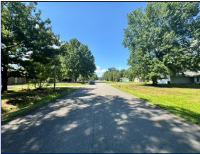
Looking N along Eve Ln
