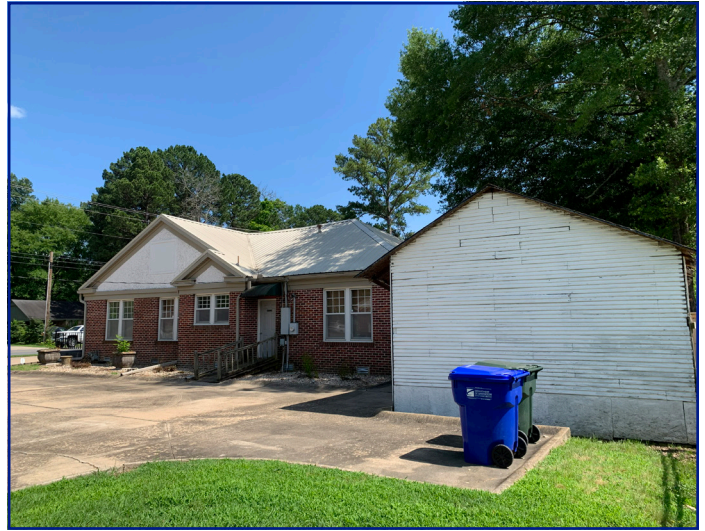
View of subject property facing SE
