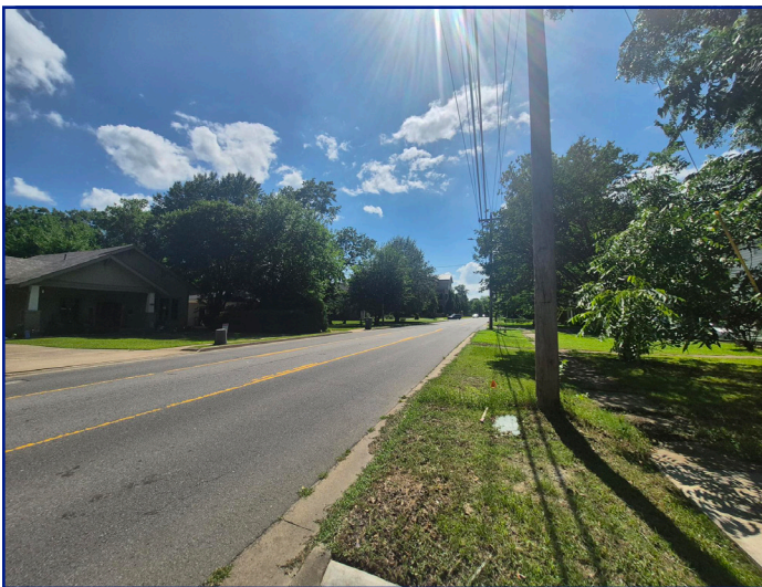
Looking W down College Ave
