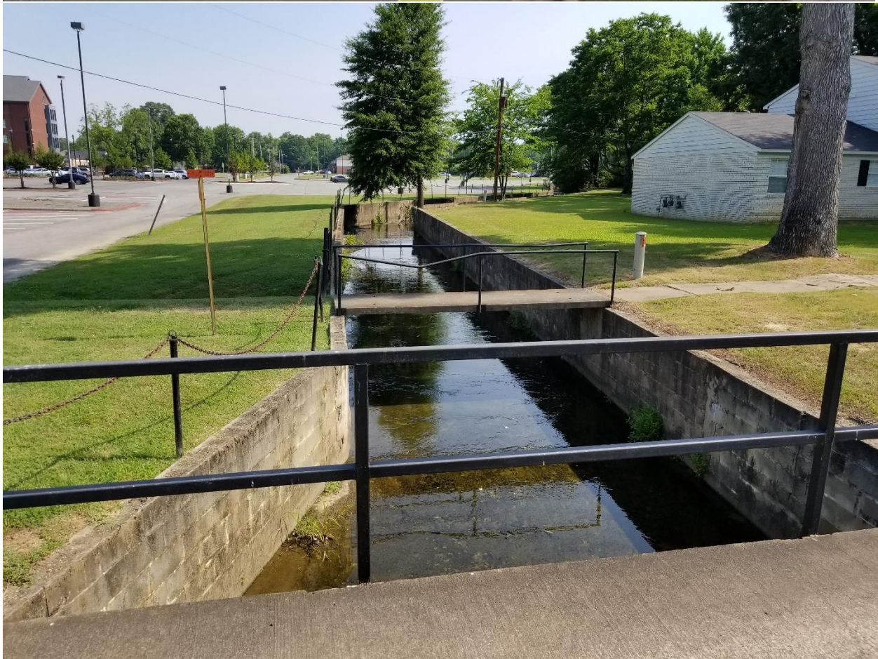
Figure 4 Site of Box Culvert to Be Installed Between Donaghey Avenue and Bruce Street
