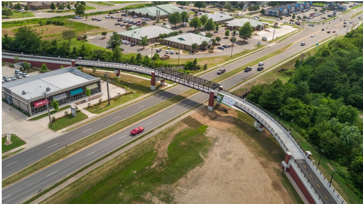
Figure 1 Newly Completed Bicycle-Pedestrian Bridge Over Dave Ward Drive
