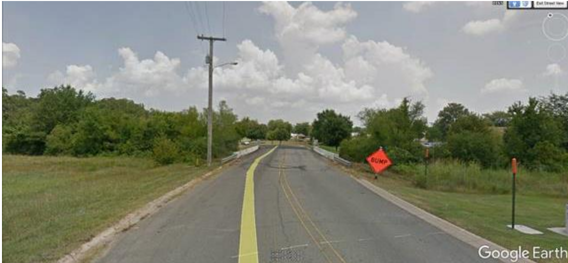
Figure 6 Bob Courtway Drive Bridge to Be Widened
