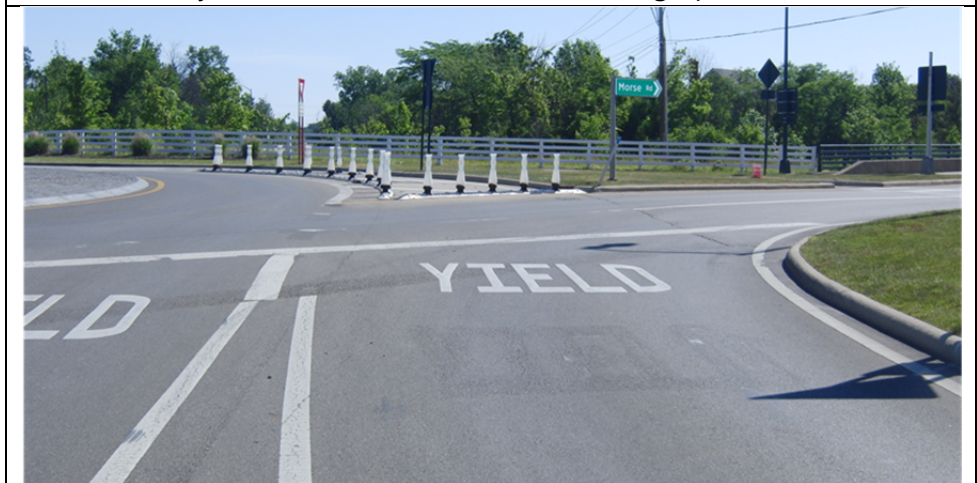
Candlestick style lane delineators with ultimate sign placement
