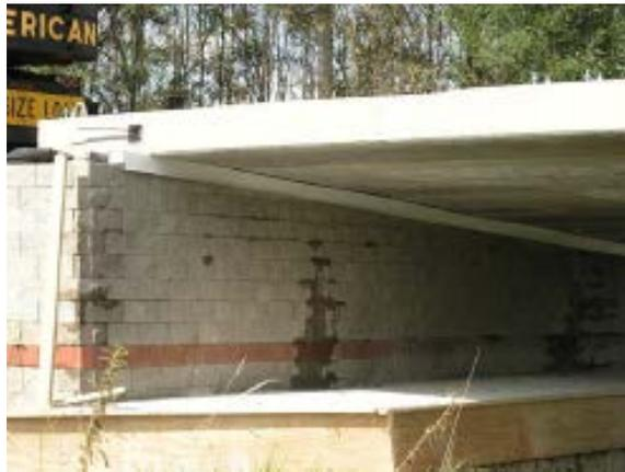
**Photo 13 - Prestressed Beams on GRS-IBS Abutment**
