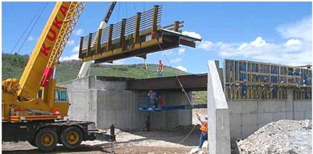
**Photo 14 - Prefabricated Steel Bridge System**
