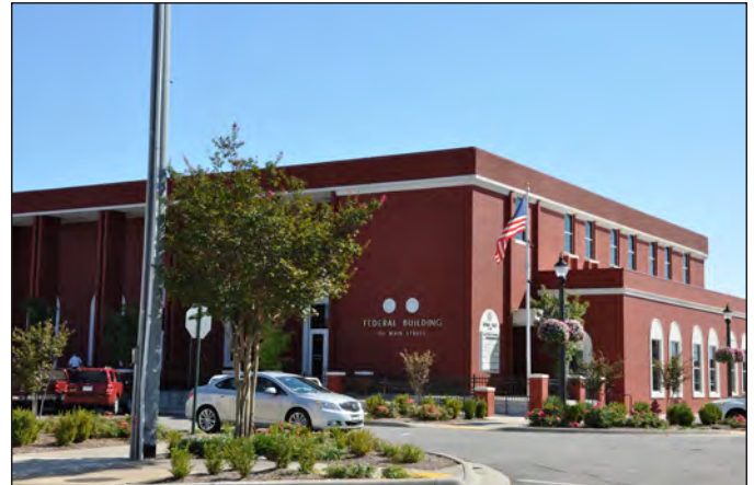
Old Post Office Building
