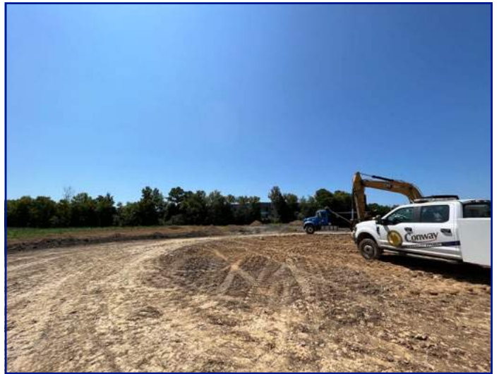
View of subject property from Central Landing PUD, looking S
