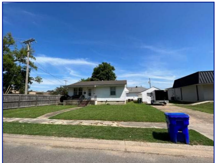
Property adjacent to the N
