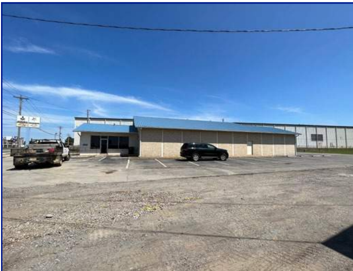
Property adjacent to the N
