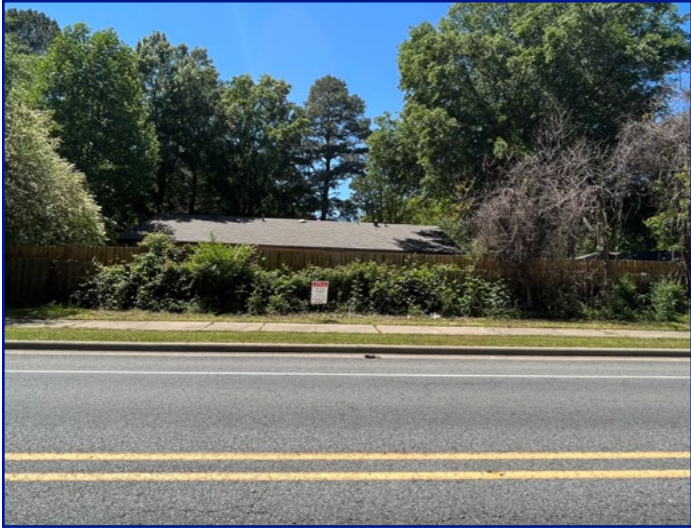
View of rear of subject property from S Farris Rd looking W
