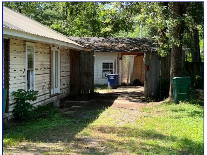
View of accessory structure at rear of subject property
