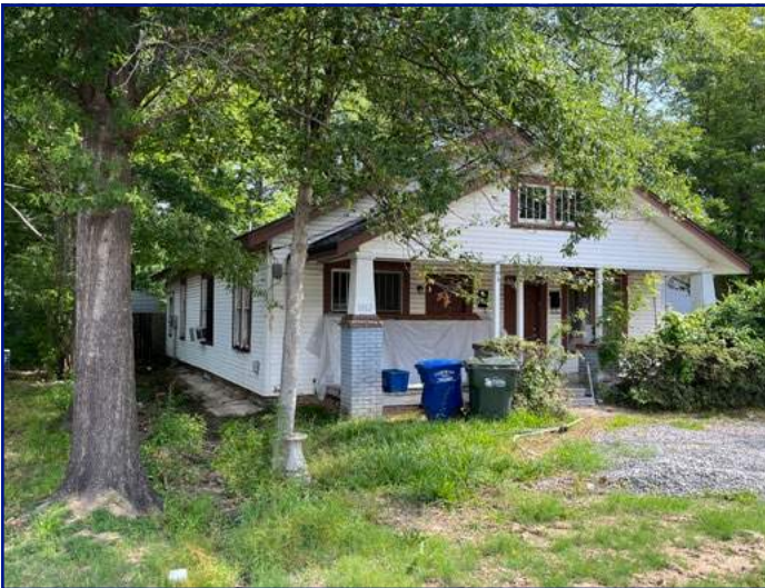
View of south and west sides of the duplex
