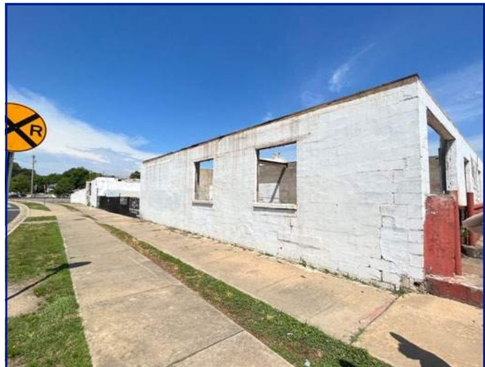
View of subject property from College Ave looking W
