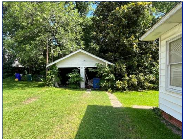
View of detached garage (to be demolished) from Prince St looking N
