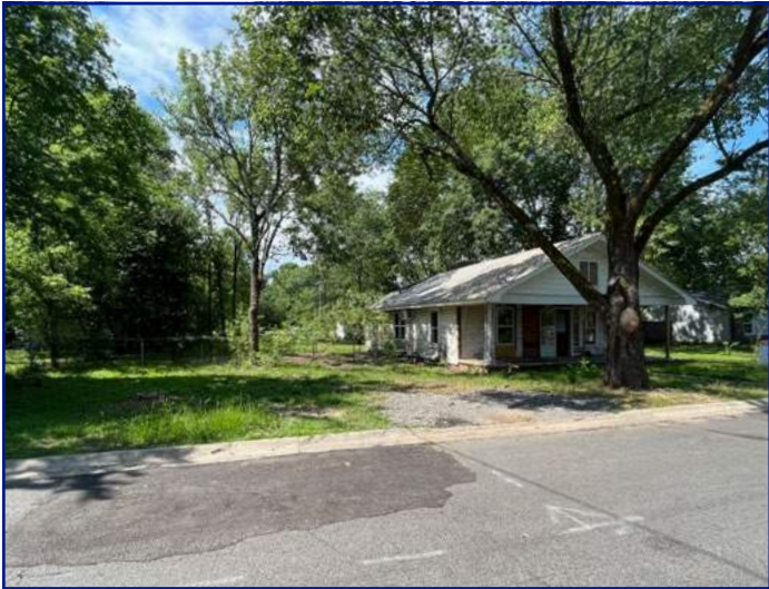
View of subject property from Hickory St looking SW
