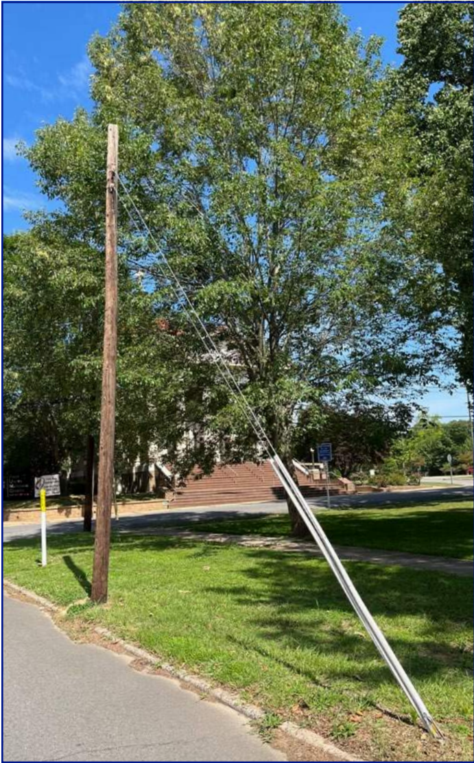
Subject utility pole at Prince St & Clifton St
