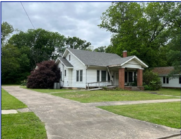
Property adjacent to the N
