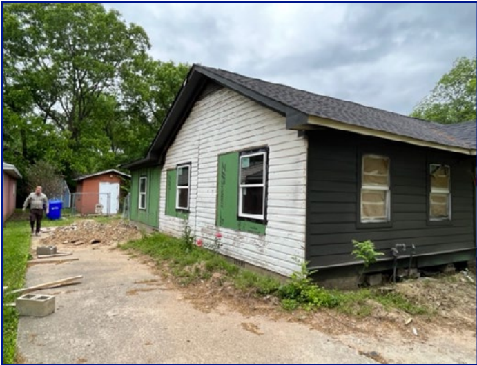
View of subject property from Locust Ave looking NW
