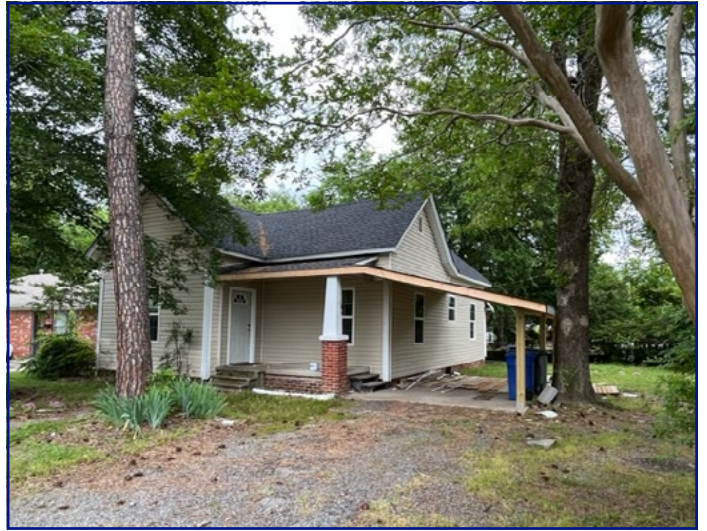
View of subject property from Watkins St looking NE
