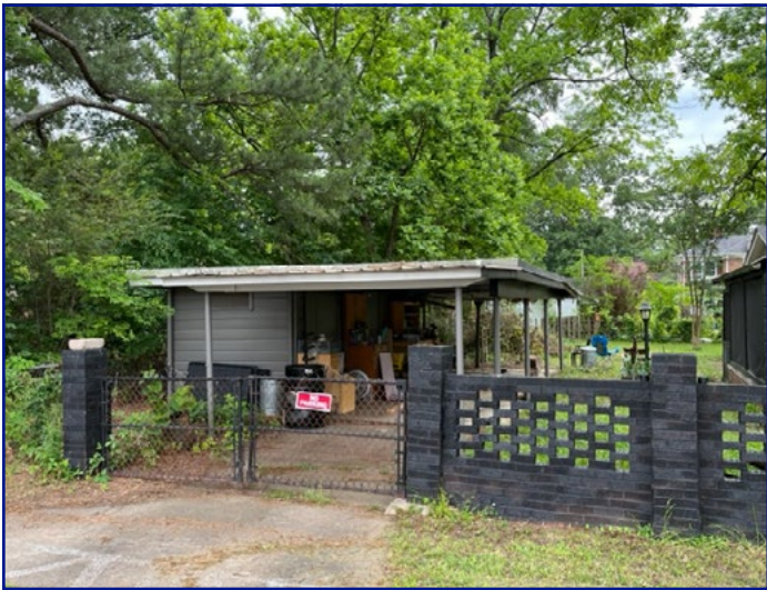
View of subject accessory structure from Cross St looking SW
