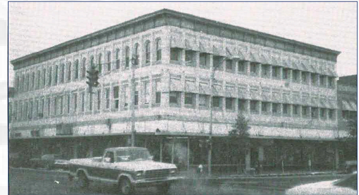
The Halter Building (c. early 1920s) [credit: Faulkner County Historical Society's Faulkner Facts and Fiddlings ]
