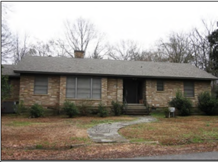
1800 JEFFERSON STREET, HENDRIX ADDITION HISTORIC DISTRICT
