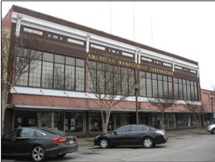
FRAUENTHAL & SONS BUILDING
