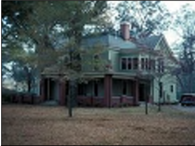
HARTON HOUSE, ROBINSON HISTORIC DISTRICT
