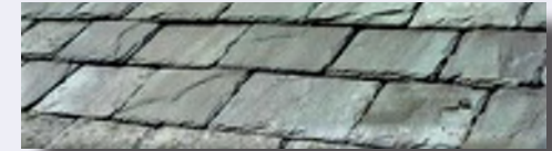
This synthetic roof has the appearance of slate.
