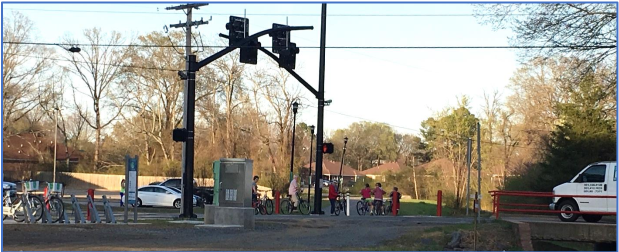
Pedestrian hybrid beacon that allows those using the Kinley Trail to safely cross Salem Road
