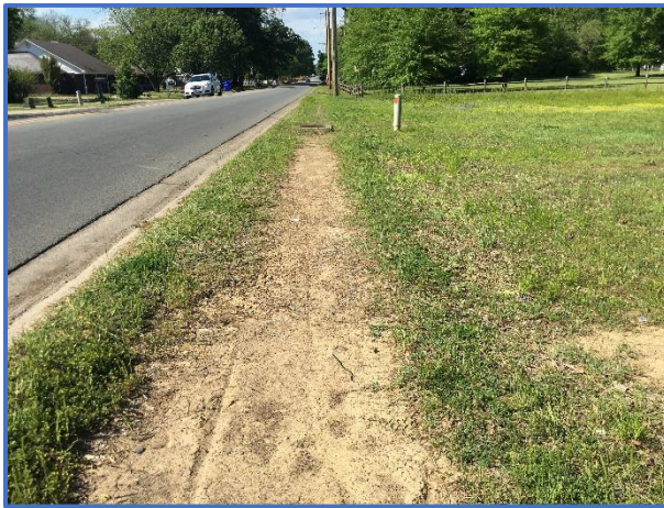
Above: Heavy foot traffic has left a path along Farris Road
