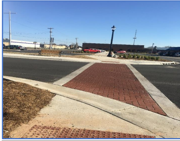
Right: Crosswalk in downtown Conway
