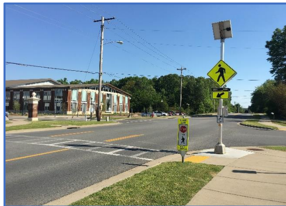
Enhanced crosswalk adjacent to UCA
