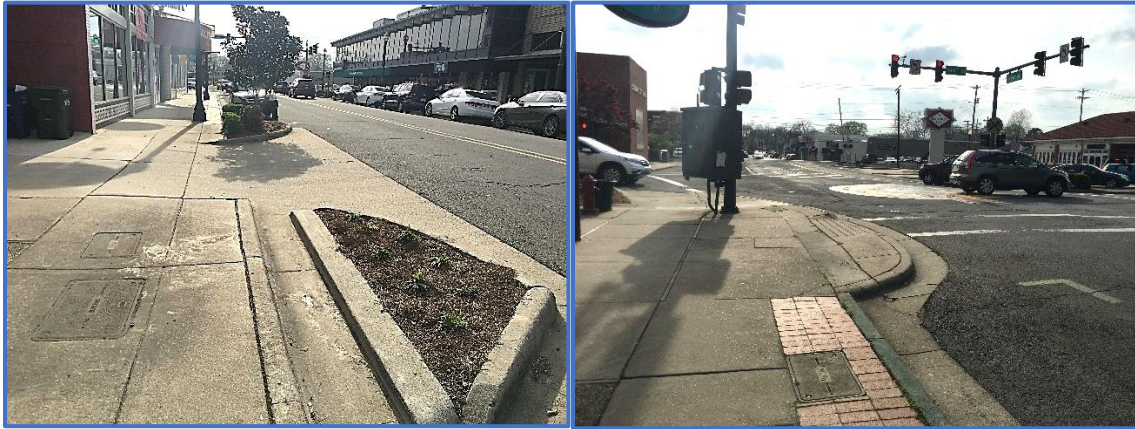
Curb extensions in downtown Conway
