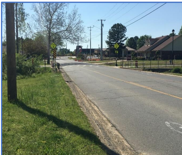
Above: College Avenue connects to many areas but lacks sidewalks
