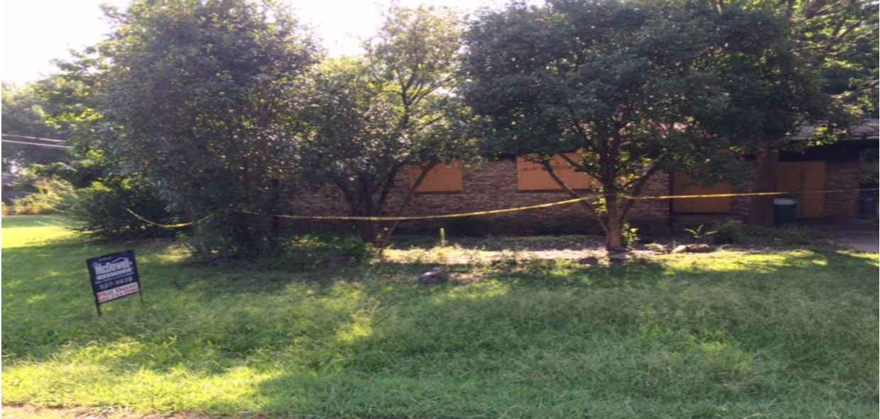
1110 Neal St. Demolition
