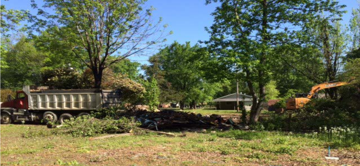
1110 Neal St. Demolition
